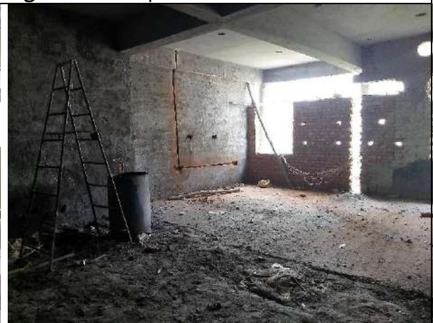
Figure 4: Under construction OT
