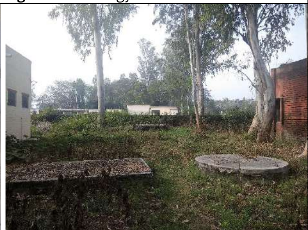
Figure 4: Bio medical waste pit
