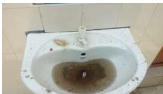
Figure 2: Toilet of Health Facility in North District, Delhi
