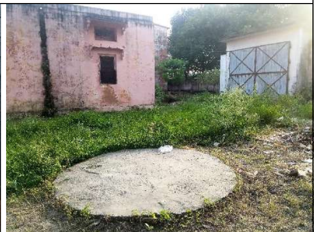
Figure F: Bio medical waste pit
