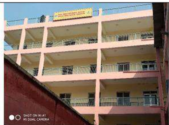
Fig: 6 Hospital Buiding, DWH, Saharanpur
