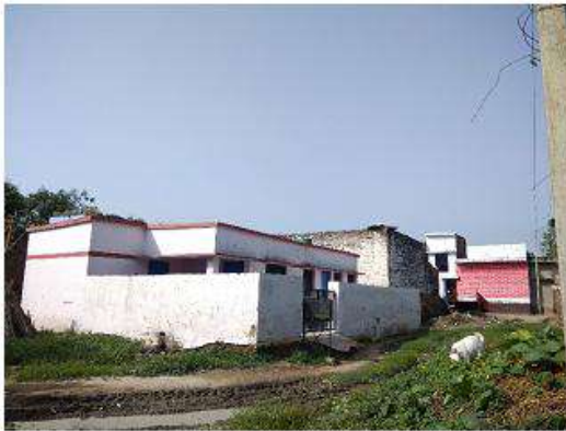
Figure 13: Sub centre, Hasanpur
