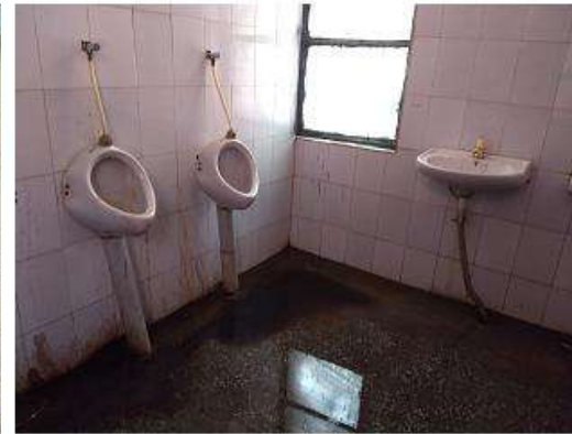
Figure 14: Water flow in bathroom, CHC, Bahjoi
