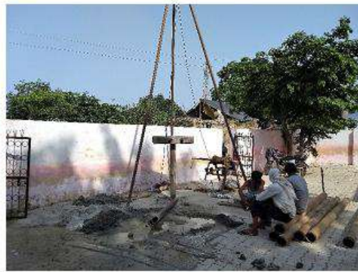
Figure 12: Bore well under construction at SC
