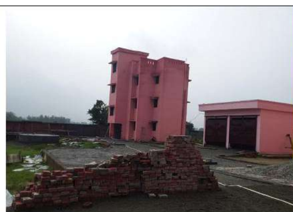
Figure 6: Under construction DH, Shamli.
