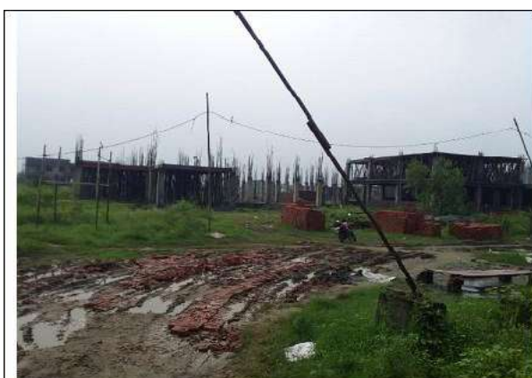
Figure 5: Under construction DH, Shamli.
