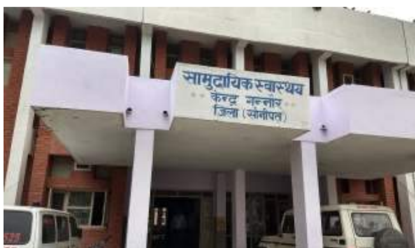
Figure 11: Community Health Centre Gannaur, Sonipat District
