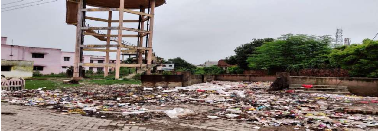
Figure 8. Waste dumping ground in the premises of DWH, Unnao
