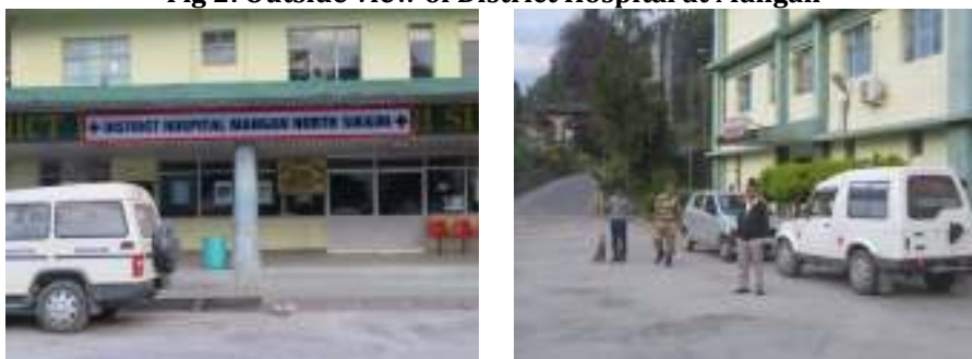
Fig 2: Outside view of District Hospital at Mangan
