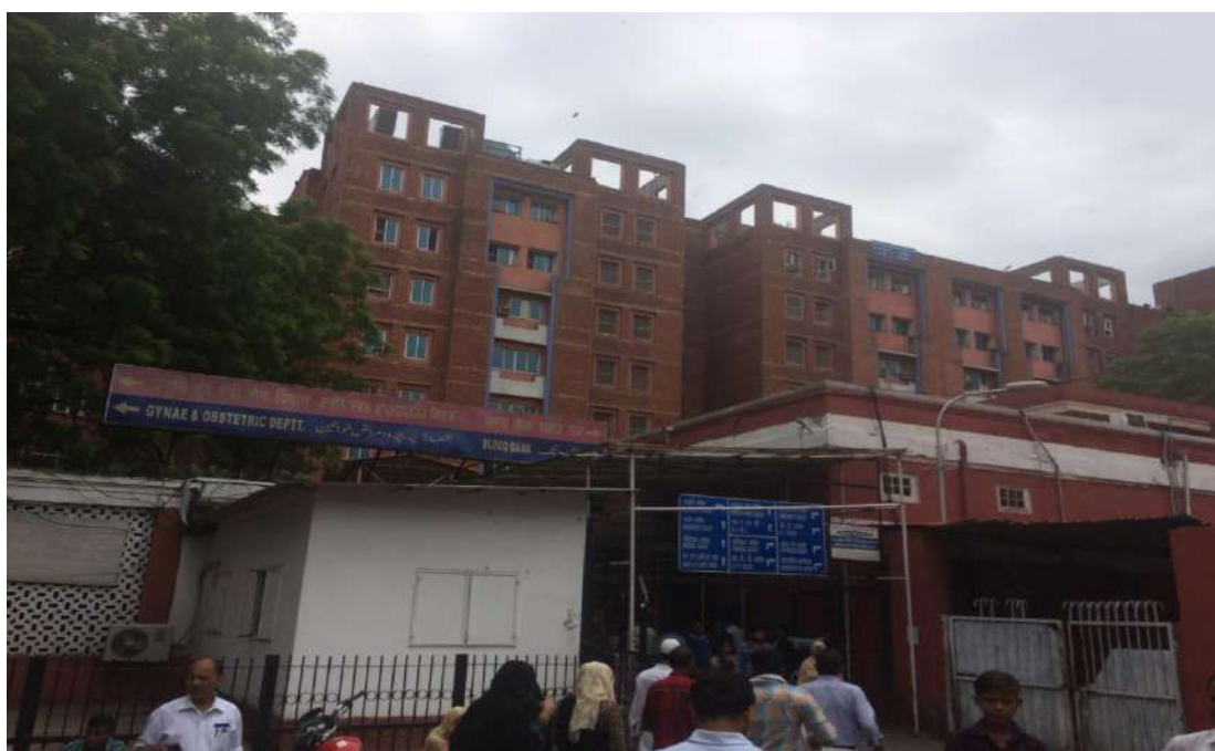
Figure 2: View of LNJP Hospital
