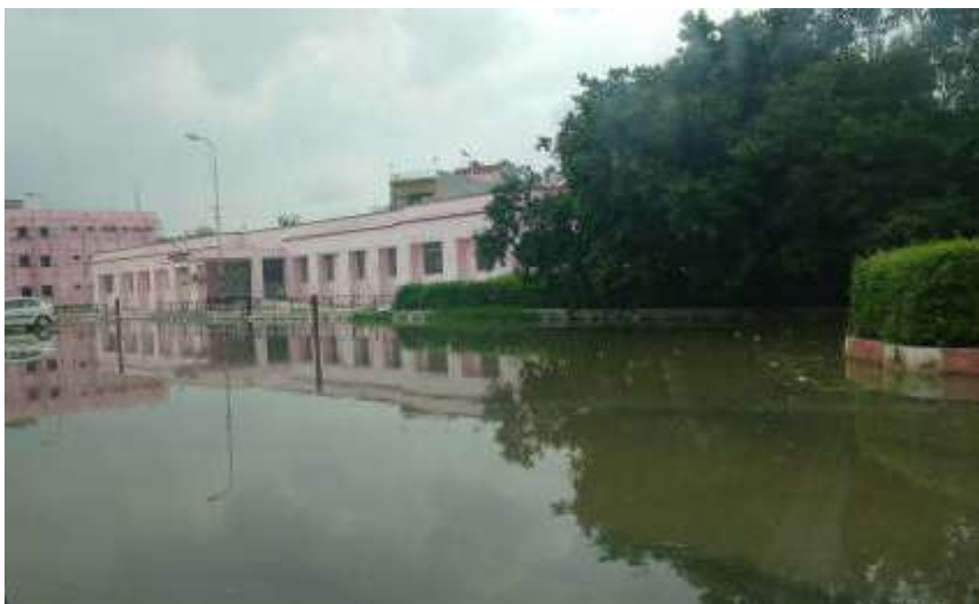
Figure 2: Waterlogging in front of CDH, Kanpur Dehat
