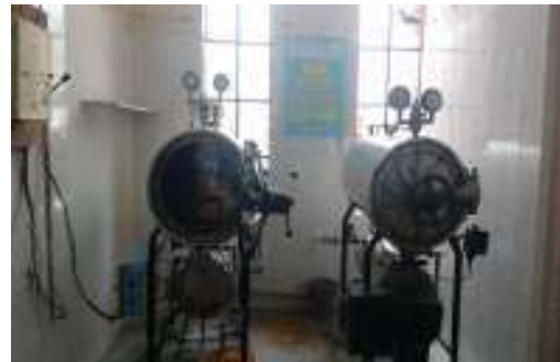
Laundry Sterilisation Room
