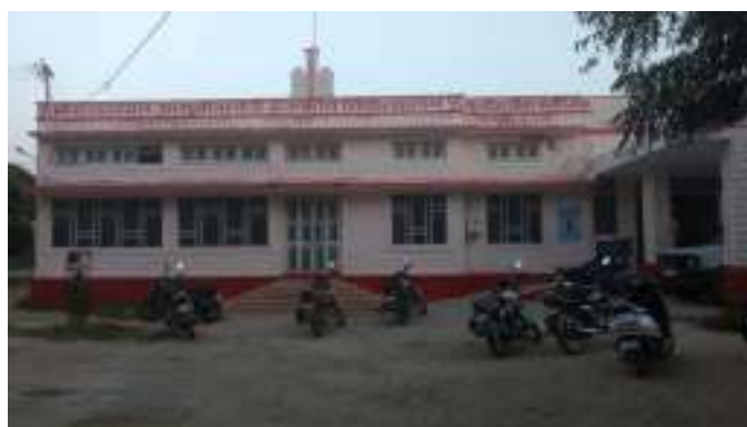
Figure 6: Primary Health Center, Gundoj Block, Pali District, Rajasthan
