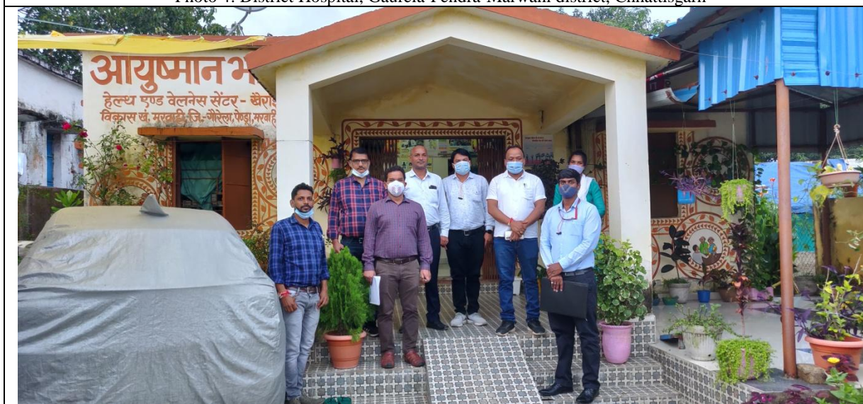
Photo 5: Sub-Centre-HWC, Khairjhiti, Marwahi block
