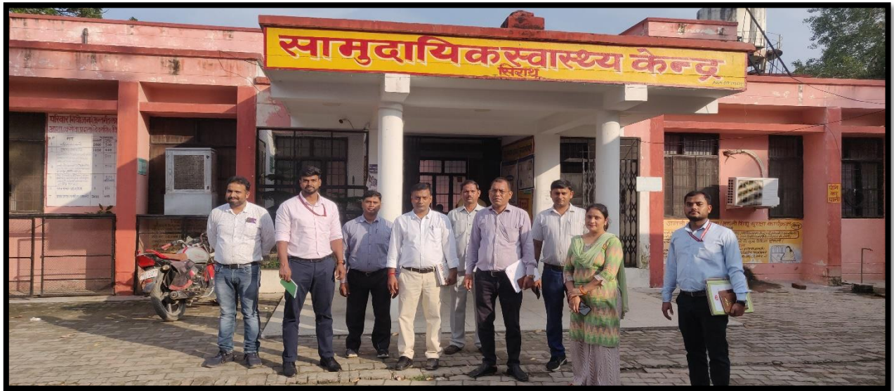
Figure 3: Community Health Centre, Sirathu, Kaushambi District
