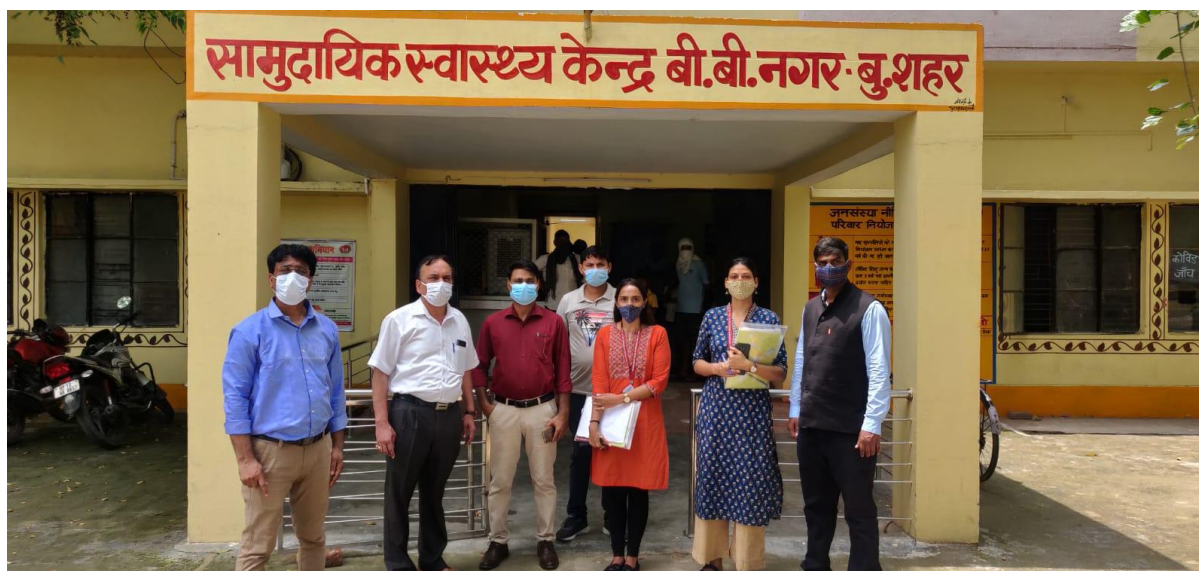
Figure 12:Community Health Centre,B.B Nagar
