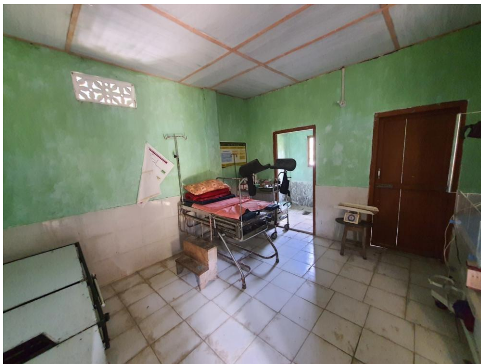
Figure 5.2: Labour Room, CHC Pakke Kessang
