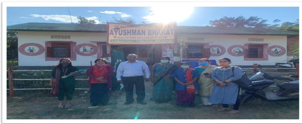
Figure 12: Sub-Centre Health and Wellness Centre,Langathel
